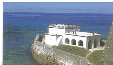
Chapel of Nossa Senhora do Baluarte (exterior and interior)
